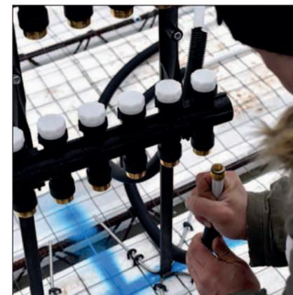
**4** RACCORDEMENT DES TUBES AU COLLECTEUR
